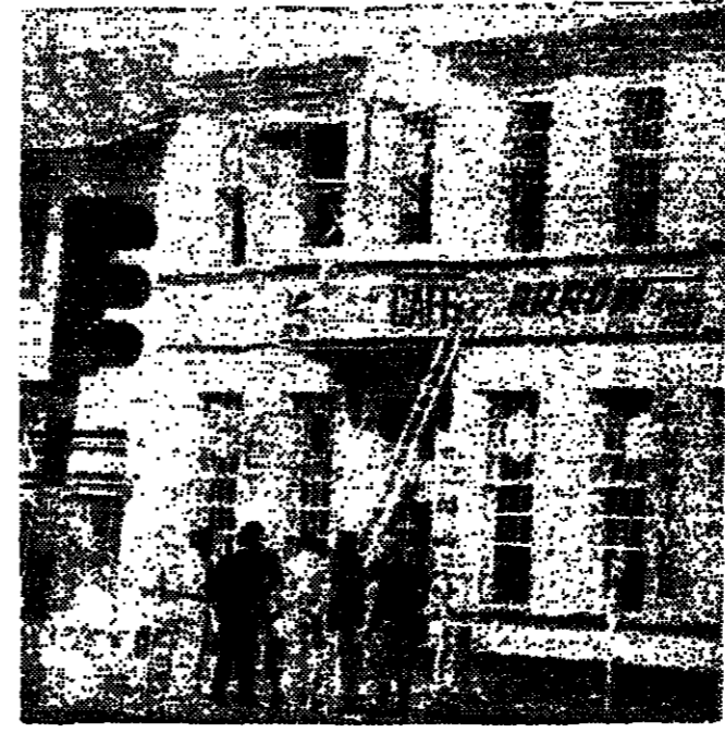
ANC office in Harare with upper windows blown out.
